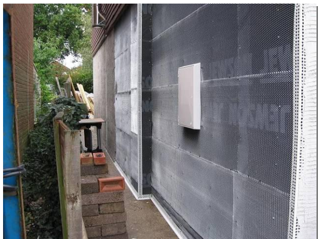
Figure 2 Insulation being applied to the walls
