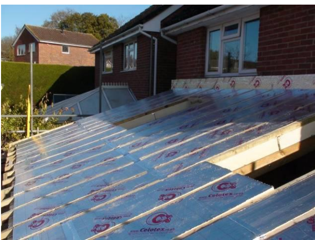
Figure 1A view of Rob's roof insulation during renovations
